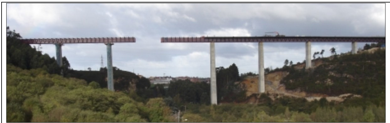
Figure 9 General view while launching
