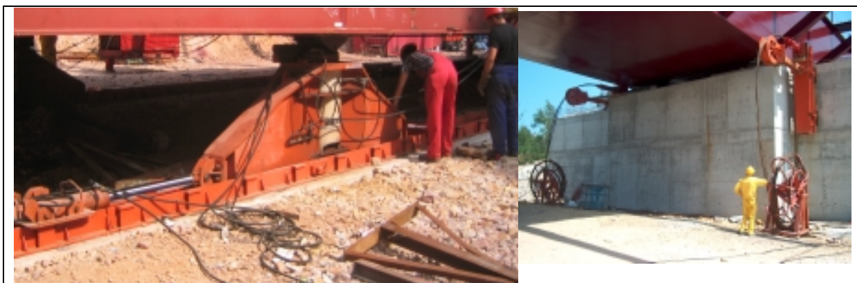
Figure 13 Pushing jacks and pulling system made of high strength steel tendons
