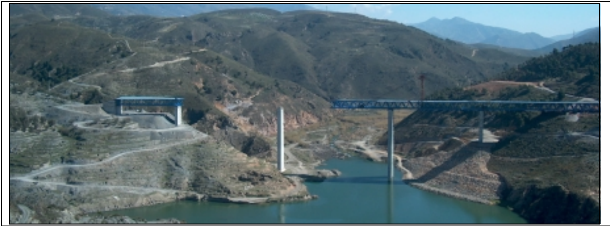
Figure 7 General view while launching
