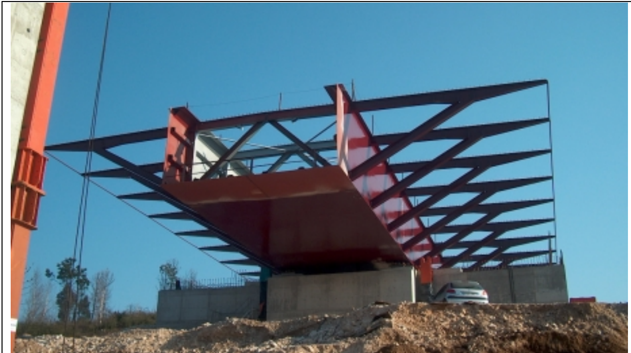
Figure 10 Cross section view while launching
