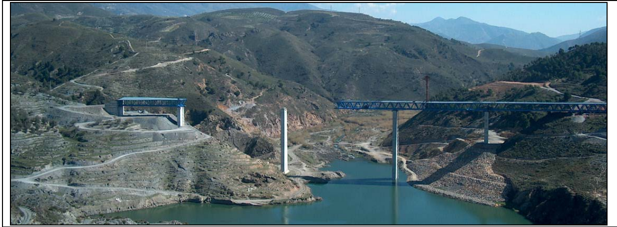
Figure 4: General view while launching
