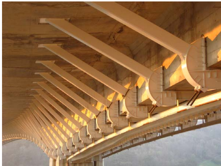
Fig. 14 Inclined steel columns to support the cantilevers.
