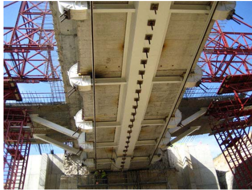
Fig. 8 Composite box section connected to the lower slab.
