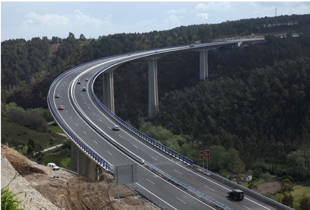
Fig. 5 The San Pedro Bridge. General view after widening the platform.
