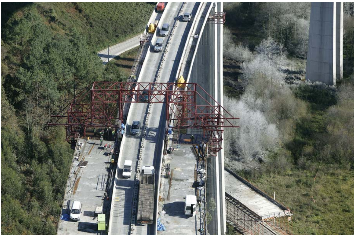
Fig. 17 Traffic on the bridge when strengthening operations were in progress using movable platform no.1
