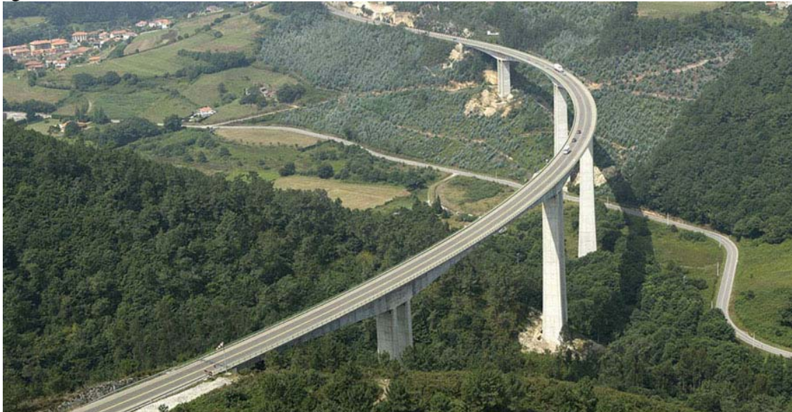
Fig. 1 General view of the original bridge
