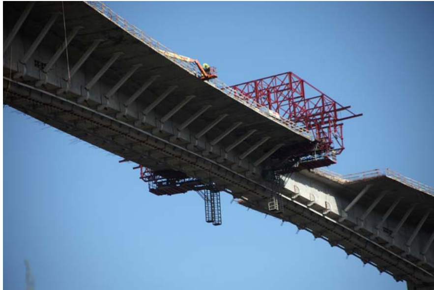
Fig. 22 New cantilevers built with platforms no. 3
