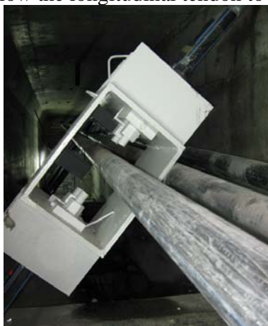
Fig. 19 Special device because of the interference of the external longitudinal tendons with the diagonal steel bars.
