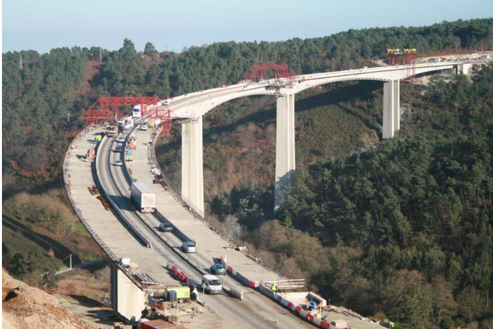
Fig. 18 General view during construction (3 movable platforms operating at the same simultaneously)
