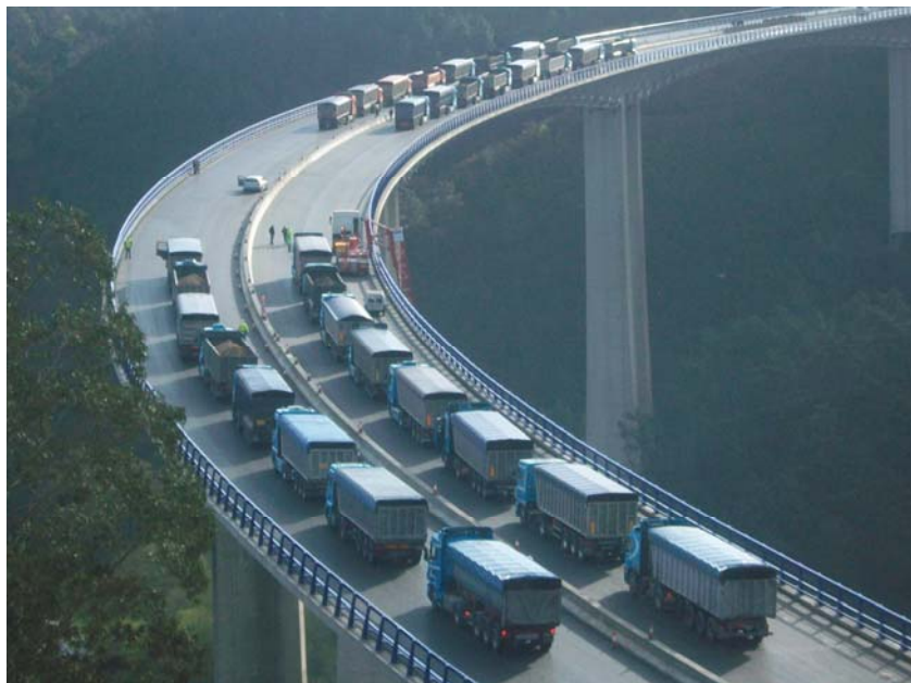
Fig. 23 General view of the widened bridge during load test
