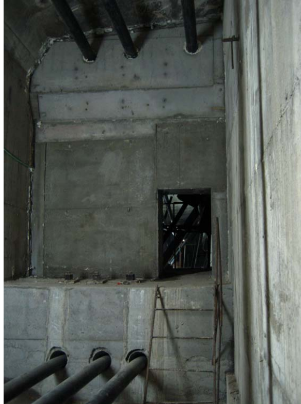
Fig. 10 Deviation walls and anchorages of the prestressing.
