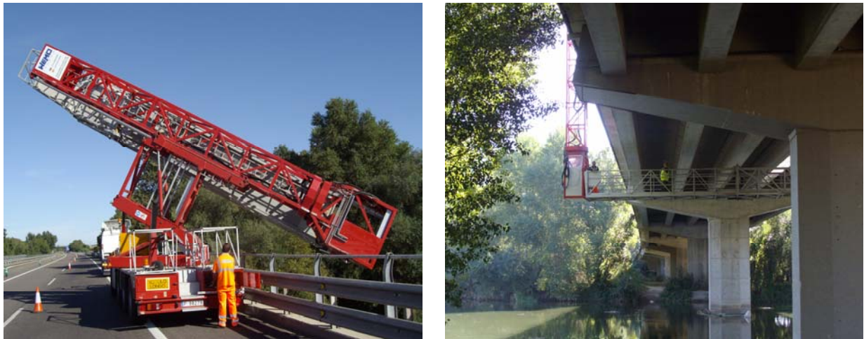
Figure 10 – General view of the self supported platform used for some inspections
