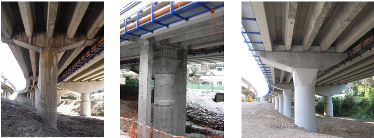
Figure 14 –Repairing works of the piers of a bridge of the AP-6
