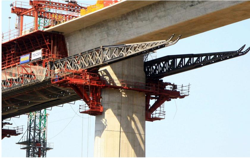
**Fig 14.** Support of the movable scaffolding of the deck on the piers
