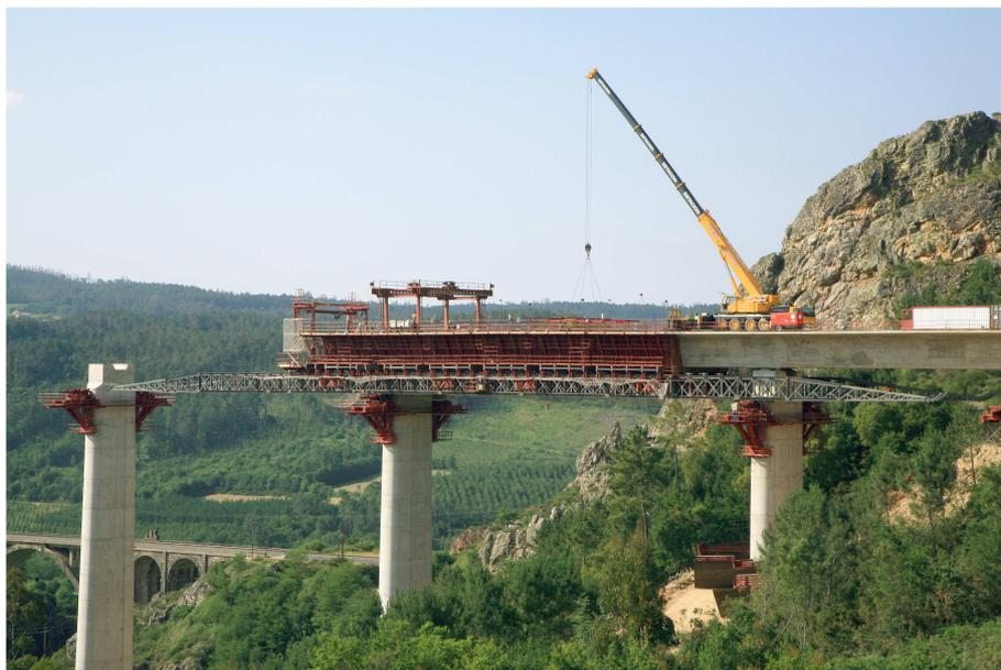
**Fig 8.** Construction of the deck
