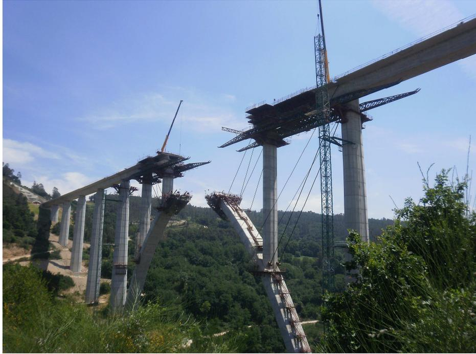
**Fig 12.** Construction of the arch
