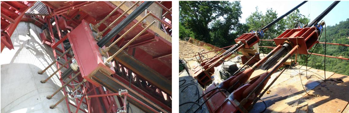
**Fig 18.** Connection of the temporary cables to the pier and to the foundation
