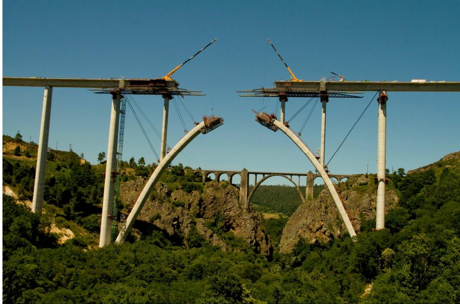
**Fig 7.** Construction of the arch
