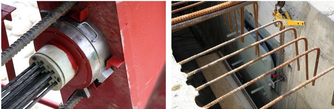
Fig 20. Load cell on temporary cable and on the longitudinal bearing of the abutment
