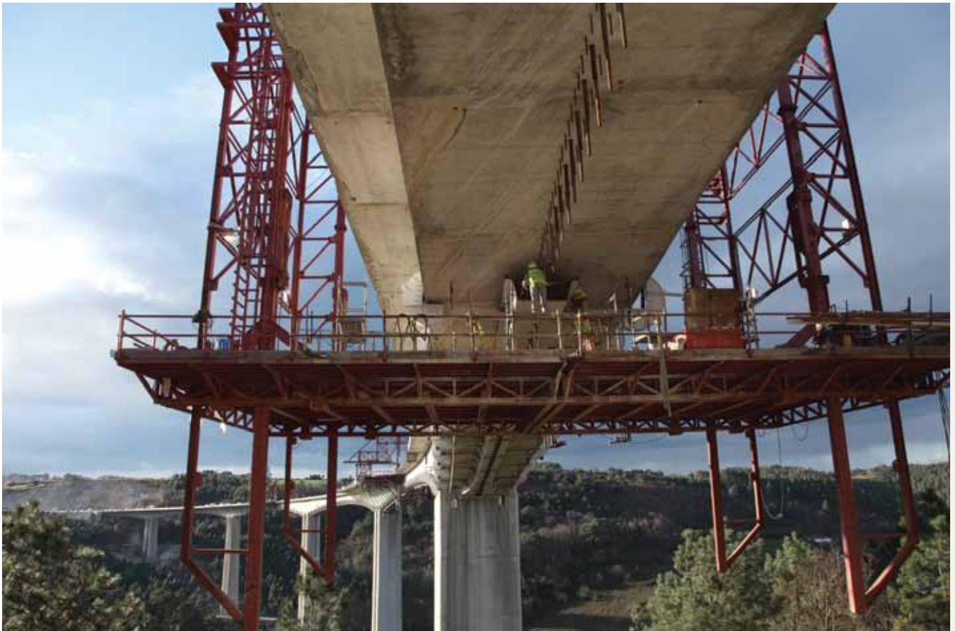
Figure 14. Composite box placed on-site using platform 1.
