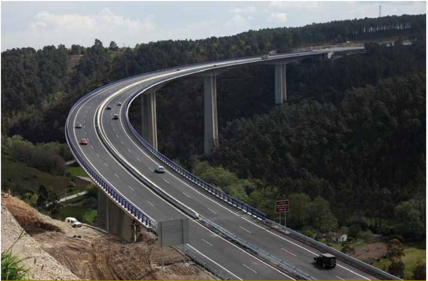
Figure 4. The San Pedro Bridge after widening the platform.
