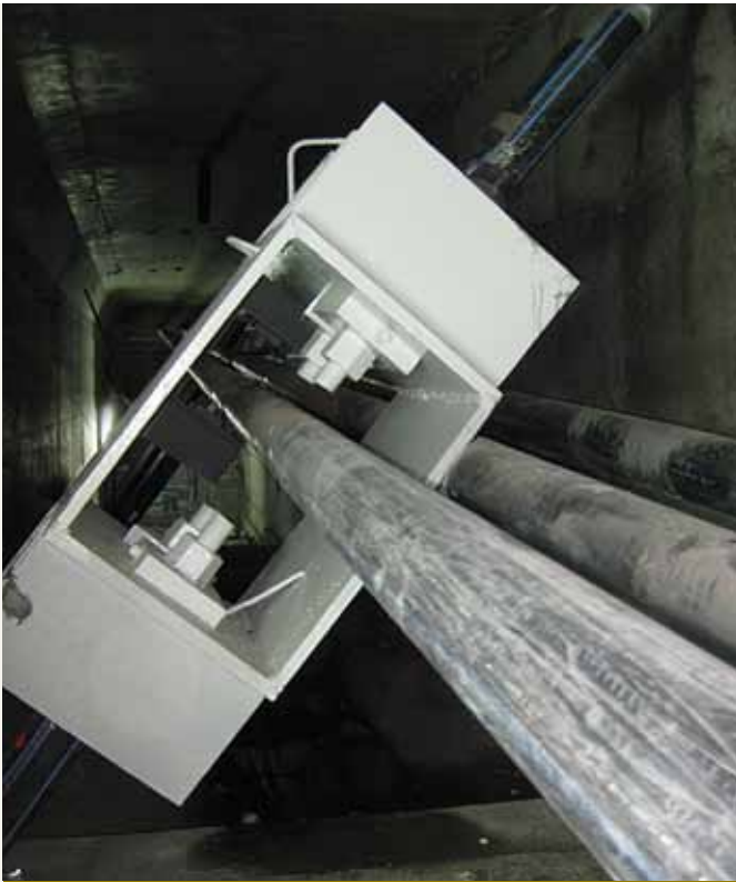
Figure 13. Special device used to eliminate the interference of the external longitudinal tendons with the diagonal post-tensioning bars.
