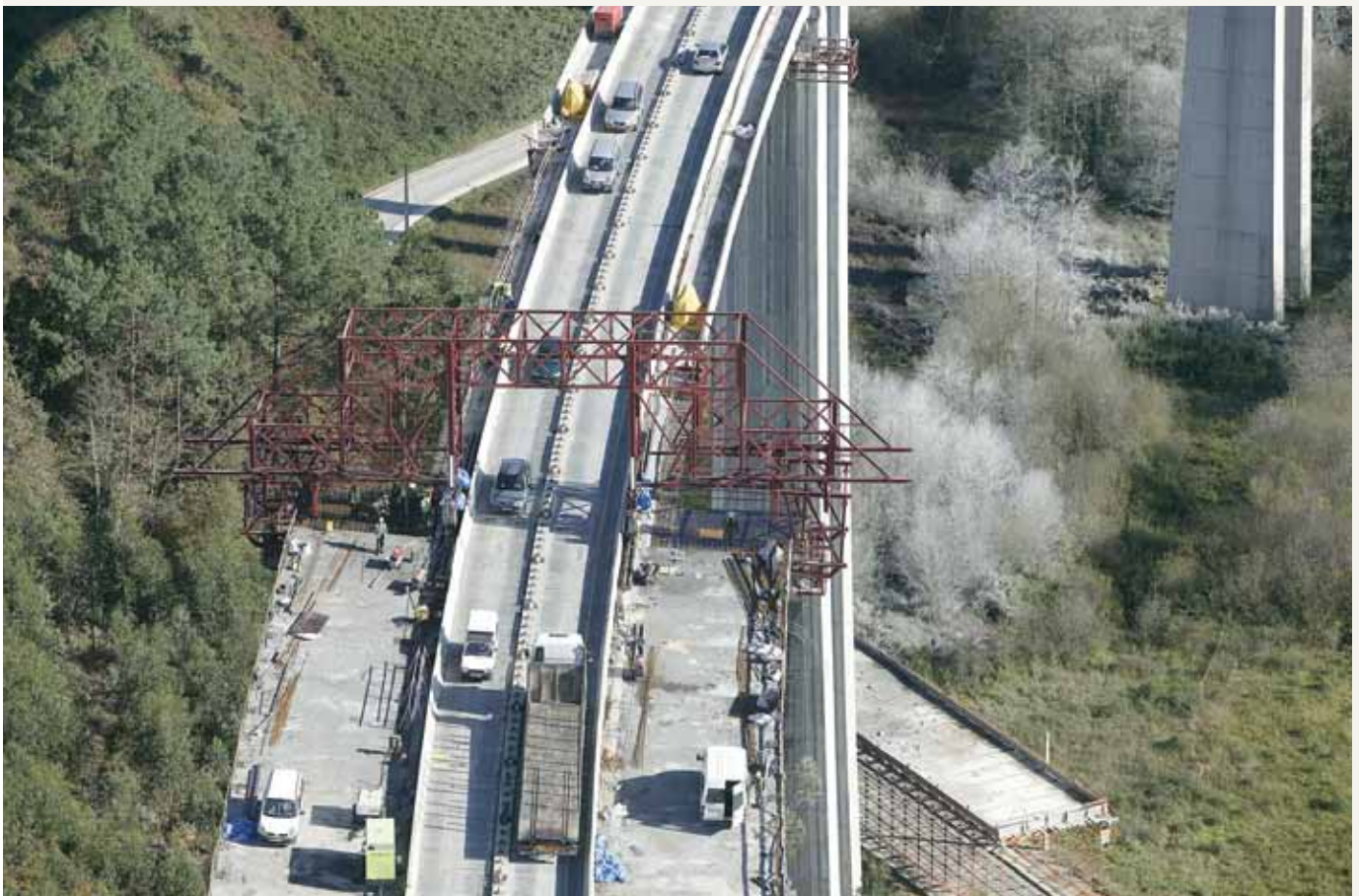
Figure 12. Traffic on the bridge using platform no. 1 when strengthening operations were in progress.
