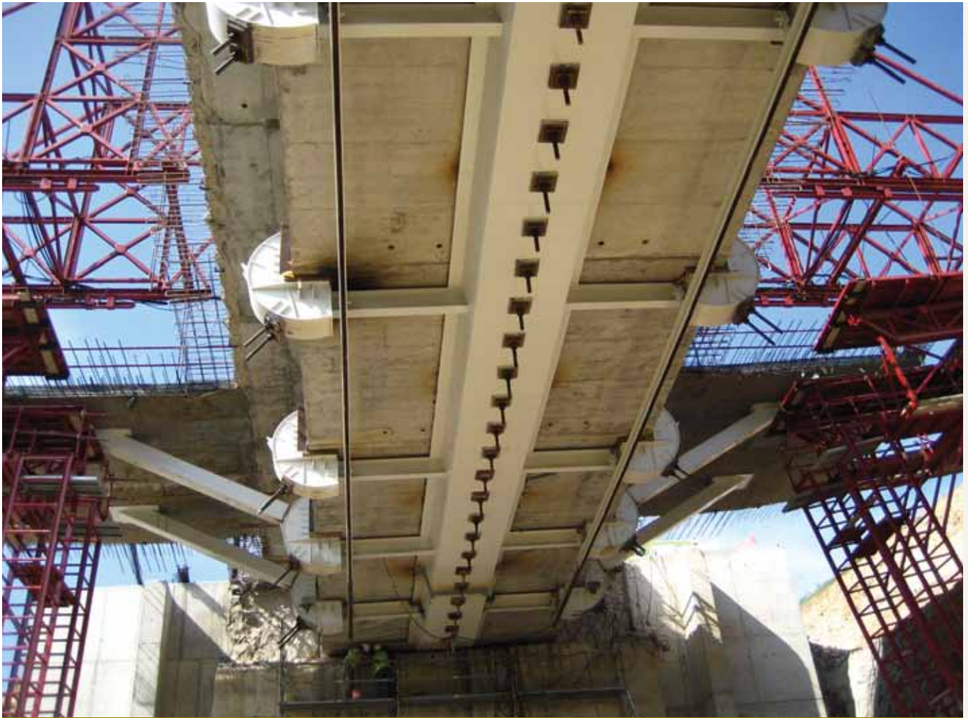
Figure 6. Composite box section connected to lower slab.
