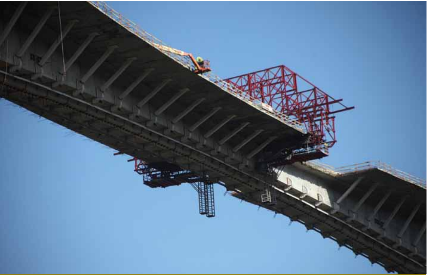
Figure 15. New cantilevers built with platform 3.
