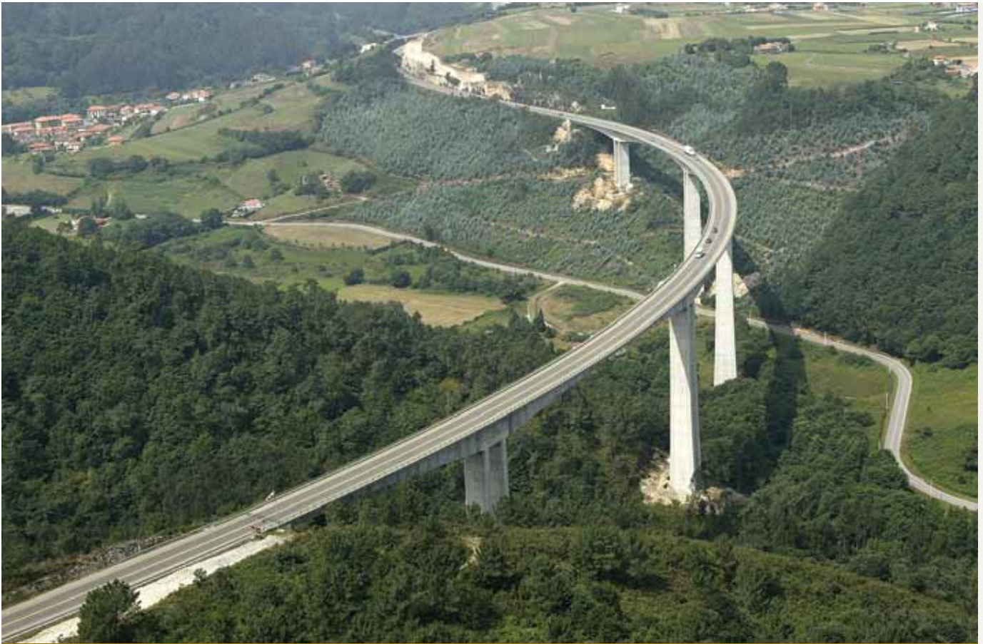
Figure 1. The original San Pedro Bridge.
