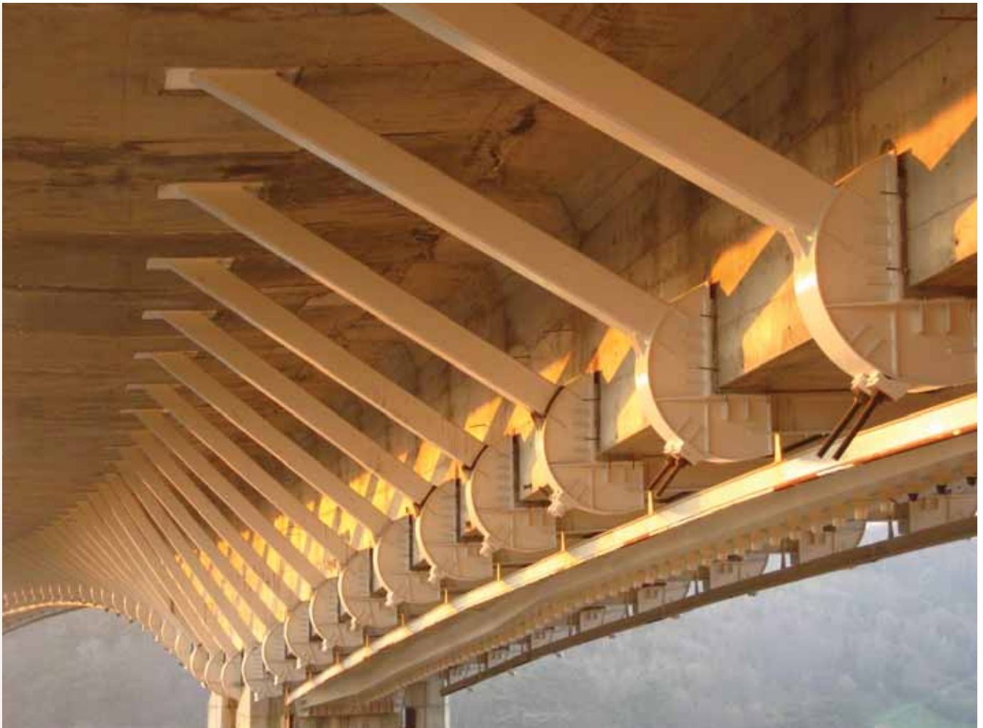
Figure 9. Inclined steel columns to support the cantilevers.
